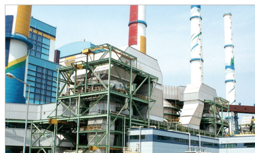
▲ Flue gas desulfurization (FGD) facilities
