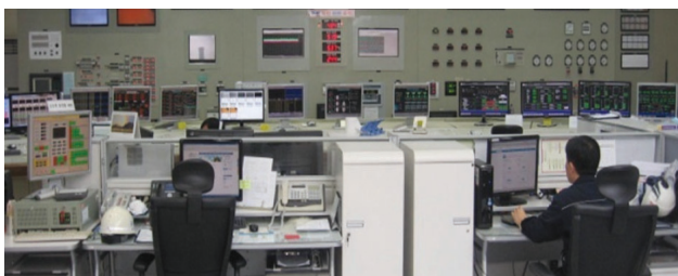
Board before replacing IMCS
