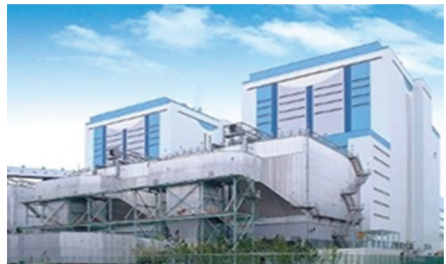
Electric precipitator
