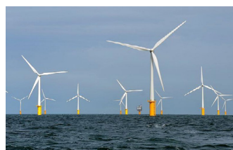
Jangbogo Offshore Wind Power
