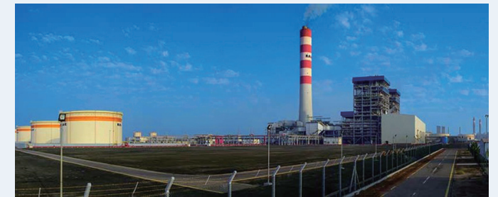
O&M for Rabigh HFO Power Plant, Saudi Arabia
