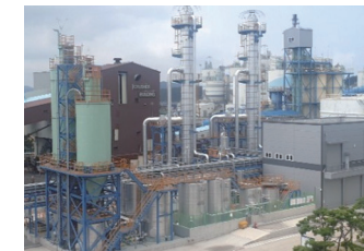
New desulfurization wastewater treatment facility (2021)
