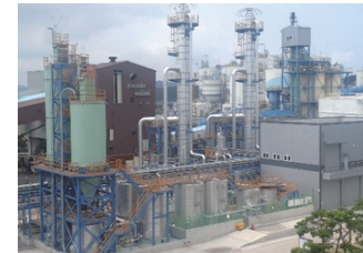
New desulfurization wastewater treatment facility (2021)
